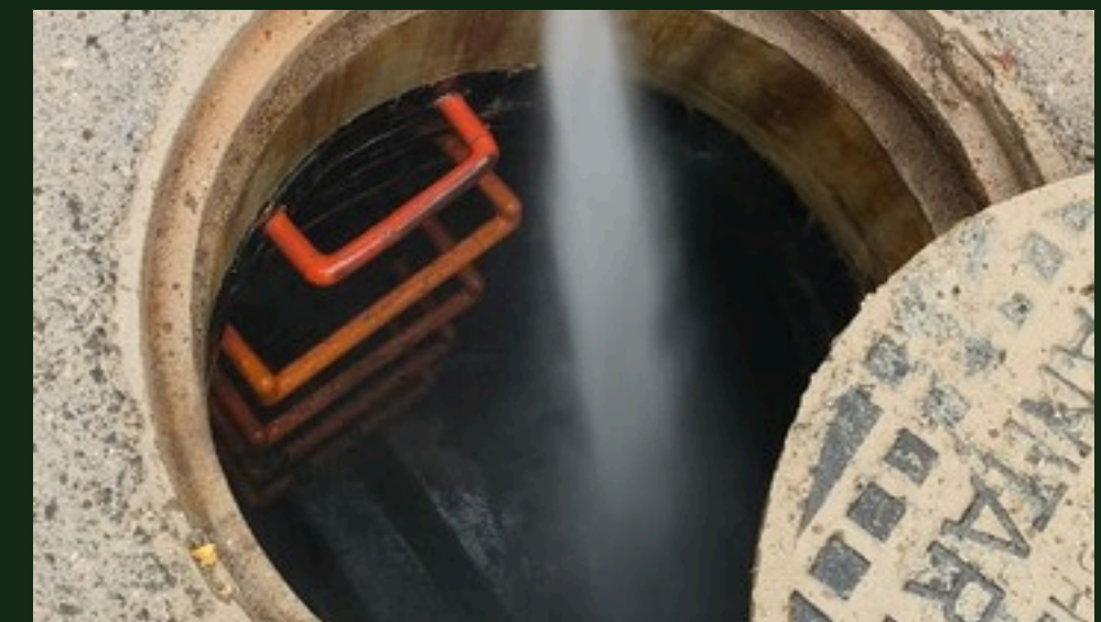
SPRAYING CHEMICAL FOR DRAINAGE SYSTEM
