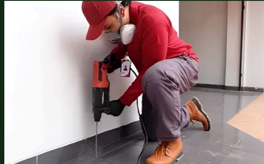
PREPARING HOLE FOR TERMITE PURPOSES
